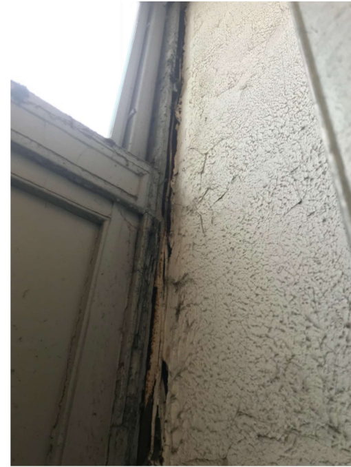
4 NORTH SIDE OF INTERIOR SPACE DATE TAKEN 11/05/2018
