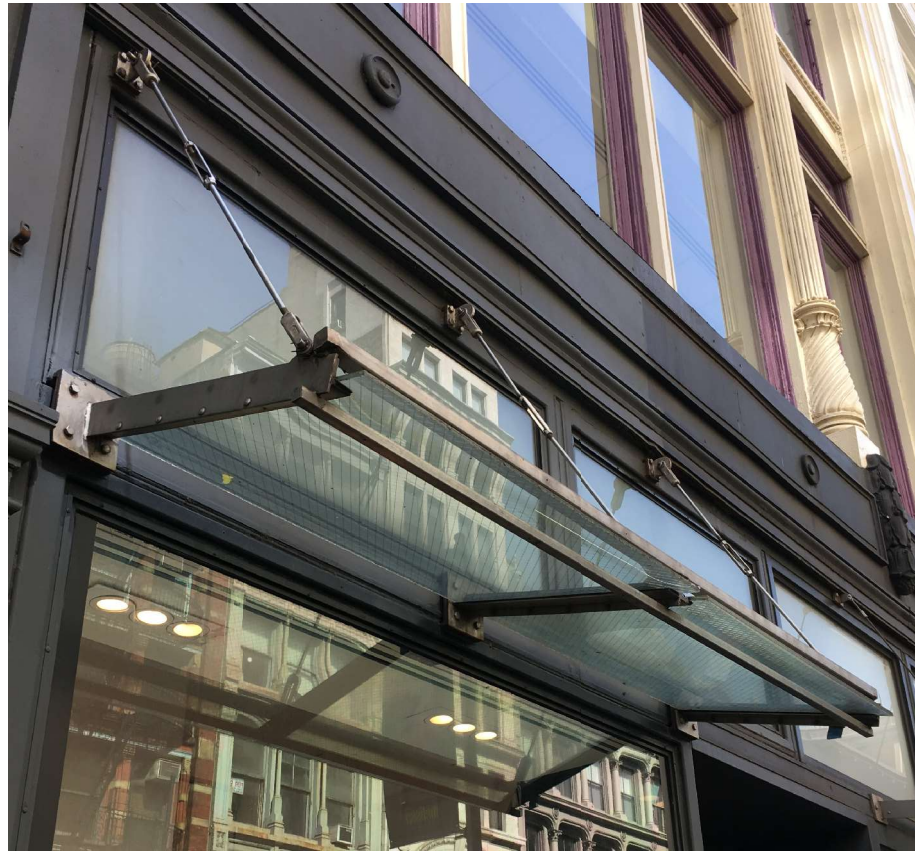
1 EXISTING AWNING OVER BANANA REPUBLIC STOREFRONT DATE TAKEN 05/03/2018
