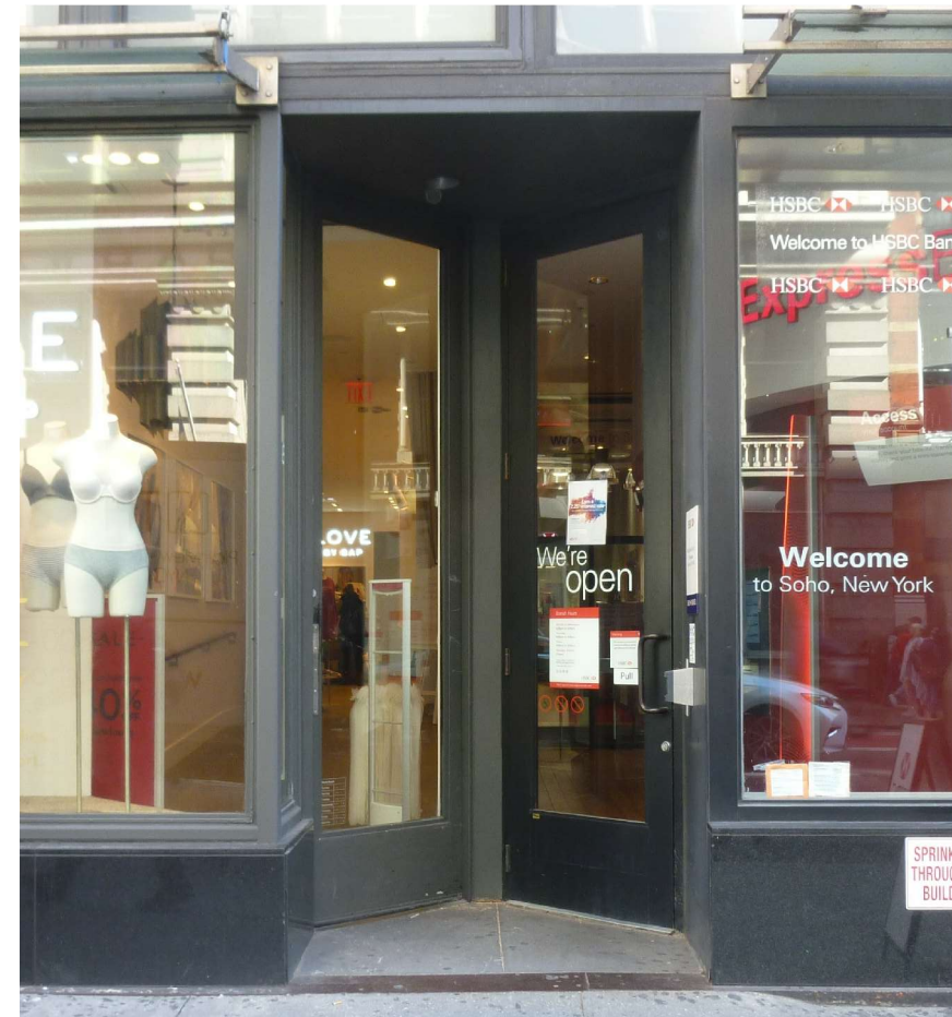
8 EXISTING BANANA REPUBLIC AND HSBC ENTRY DOORS DATE TAKEN 10/17/2018
