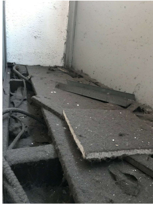
2 INTERIOR SPACE BEHIND WOODEN PANEL EXISTING ELECTRICAL WIRES AND DEBRIS AT BOTTOM PORTION
