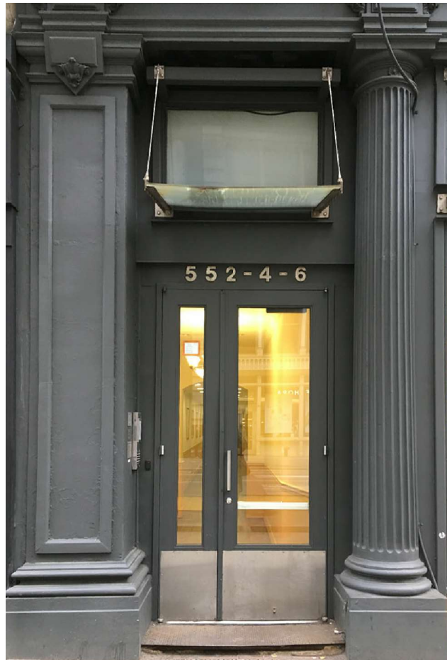
6 ADJACENT BUILDING ENTRY, 552 BROADWAY DATE TAKEN 04/17/2018
