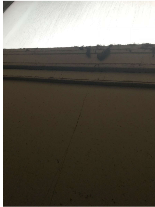
3 INTERIOR SPACE BEHIND WOODEN PANEL LOOKING UP TOWARDS TRANSOM BAR AND TRANSLUCENT TRANSOM WINDOW
