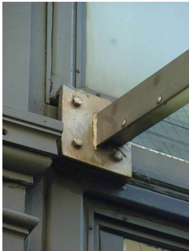
3 BOTTOM AWNING CONNECTION AT EXISTING TRANSOM BAR DATE TAKEN 10/17/2018
