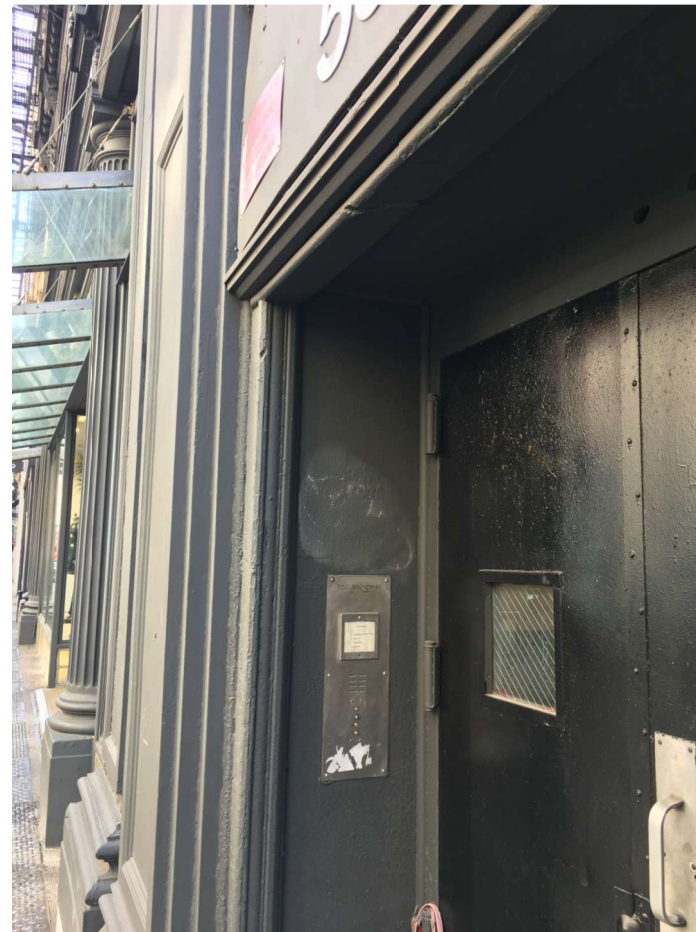
7 NORTH SIDE OF BUILDING ENTRY DATE TAKEN 05/03/2018
