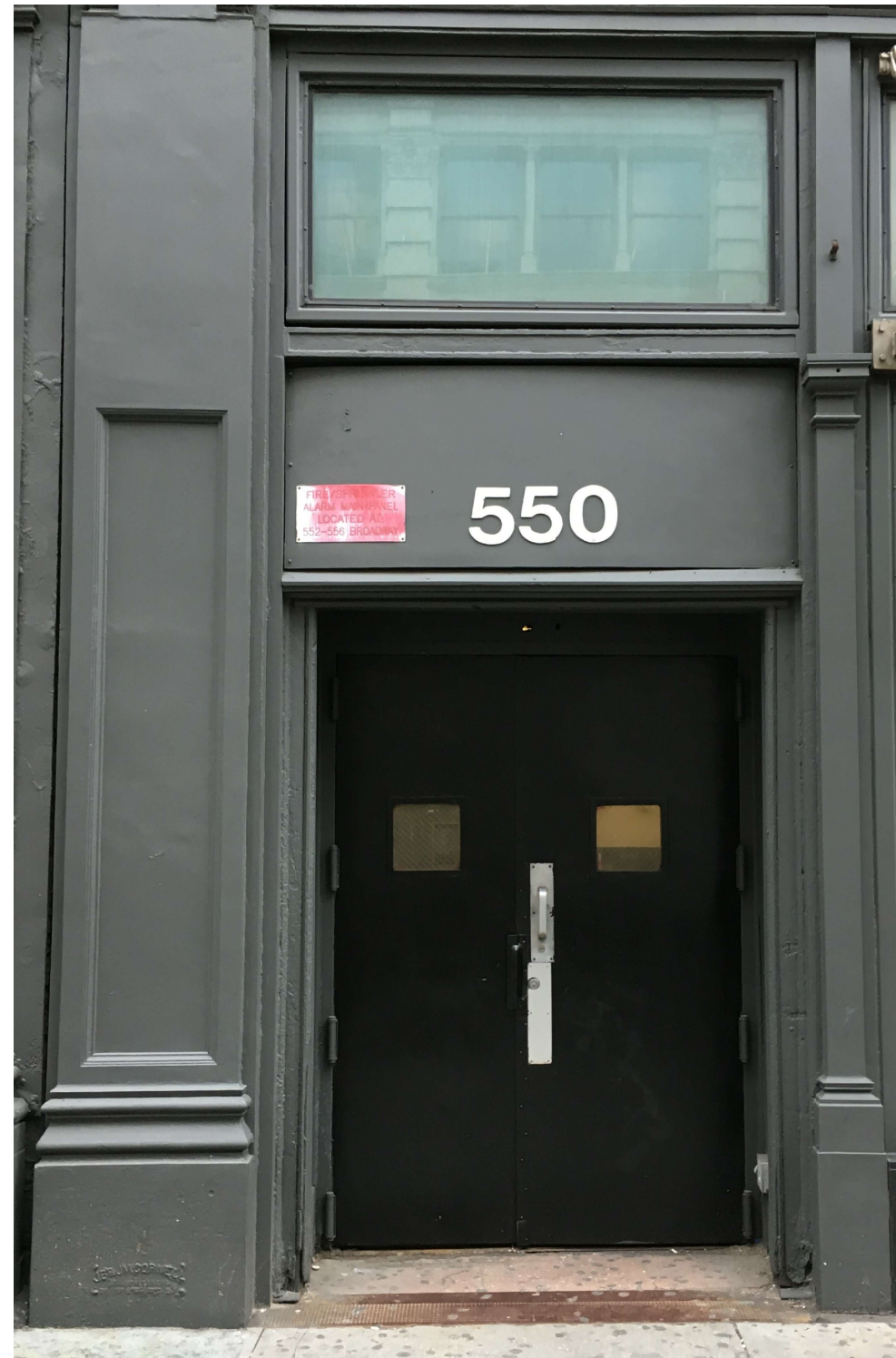
1 EXISTING NORTH DOOR BAY DATE TAKEN 05/03/2018
