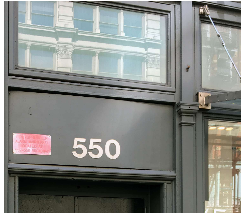
2 EXISTING TRANSOM BAR, PROPOSED AWNING LOCATION DATE TAKEN 05/03/2018
